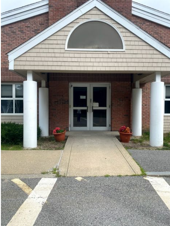
2nd grade and 3rd grade Entrance/Exit
